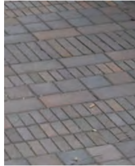
Mixed format brick feature paving
