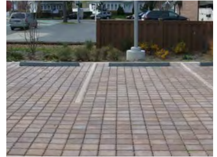
Permeable paving
